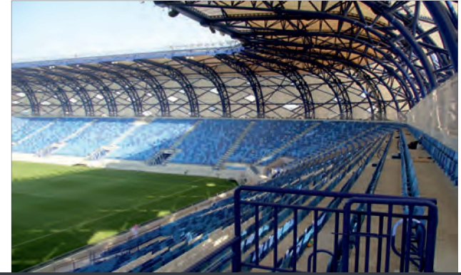
Al-Maktoum Stadium / Dubai
